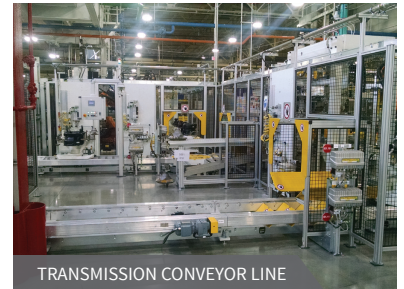
TRANSMISSION CONVEYOR LINE
