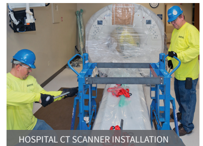
HOSPITAL CT SCANNER INSTALLATION
