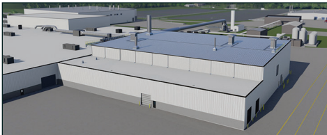
Kenworth's Chassis Paint expansion is expected to last well into 2025.
