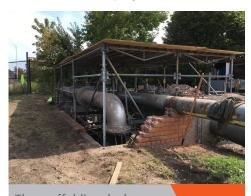
The scaffolding deck constructed above the gas pipe kept the property safe during demolition.
