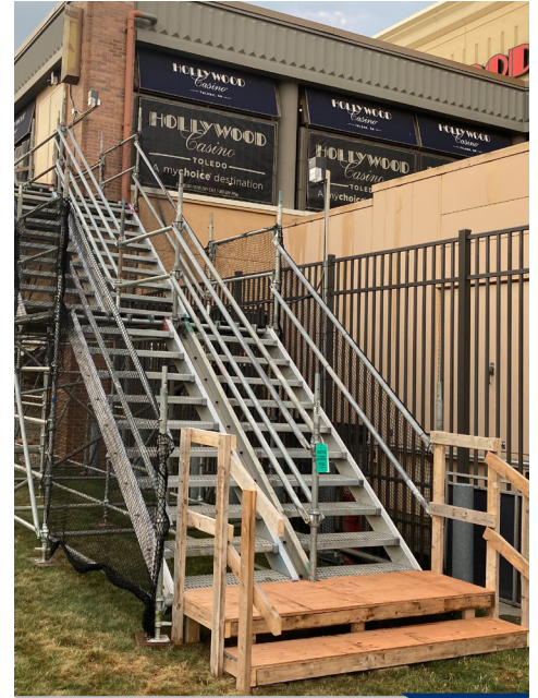
The casino egress stairway
