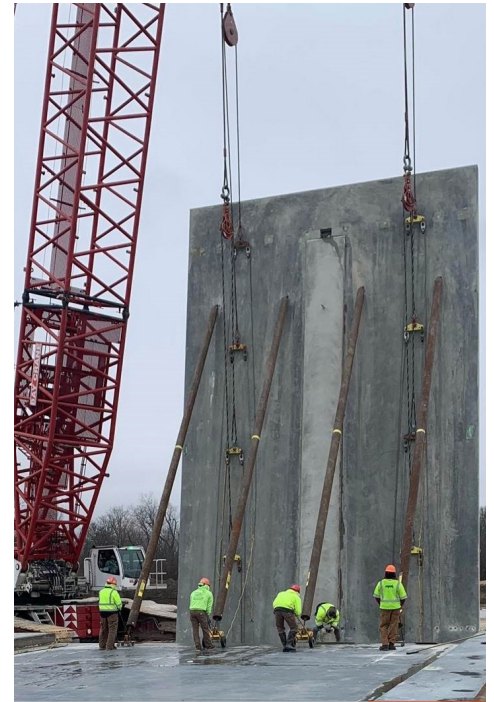
The largest, heaviest panel being lifted into place
