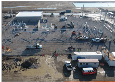
The First Solar substation is under construction.
