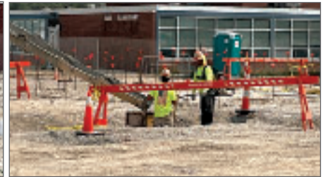
Millbury – RLI brick masons lay the first course of perimeter block, left, while a carpenter and cement finisher work on piers at the Lake Elementary School construction site.
