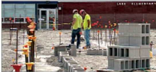
Millbury – RLI brick masons lay the first course of perimeter block, left, while a carpenter and cement finisher work on piers at the Lake Elementary School construction site.
