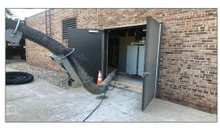
Above: The long vacuum hose eliminated the need to dig by hand. Right: The tree roots exposed by the hydro-excavator.
